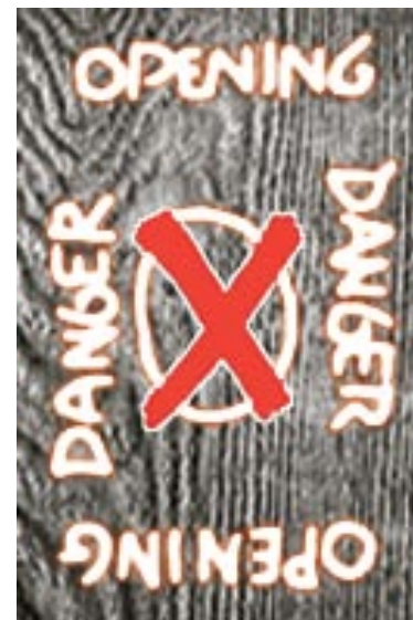
Example of markings on a plywood cover.
