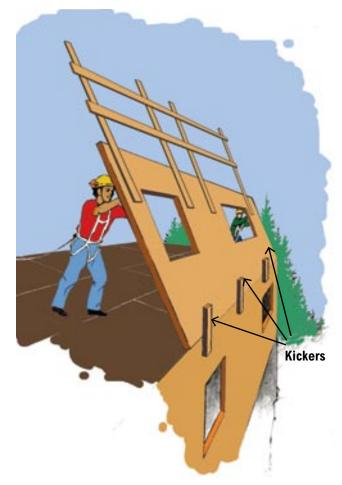
Install kickers to prevent the bottom of the wall from slipping off the subfloor. In addition, guardrails can be nailed prior to lifting to deter walking the top plates and to provide fall protection to workers on the next level.
