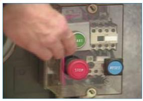
Test the lockout by pressing the start button.
