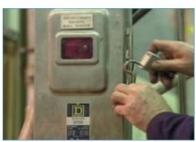
After disconnecting the machine from the electrical source, apply a personal lock.
