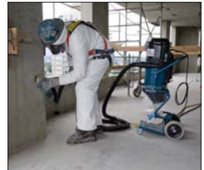
Worker grinding concrete using local exhaust ventilation
