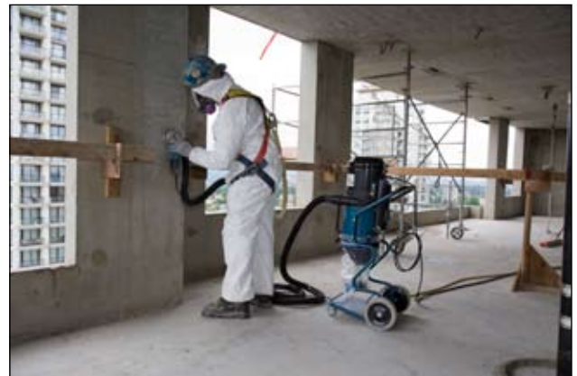
Wall grinding with LEV
