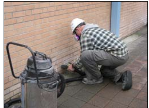
Tuckpoint grinding with LEV
