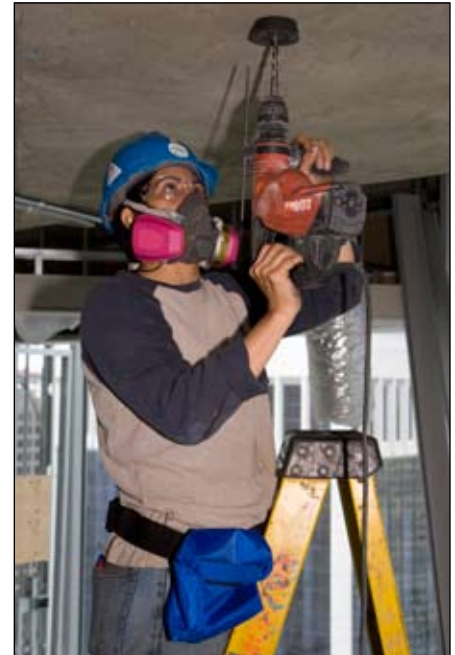
Drilling using a dust cap
