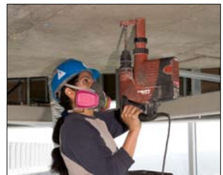
Drilling using a dust cap
