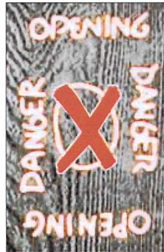
Examples of markings on a plywood cover.
